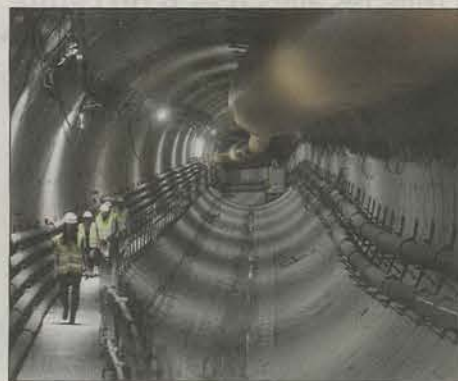
Le tunnelier approche Victor-Hugo. (Photo archives NM)
